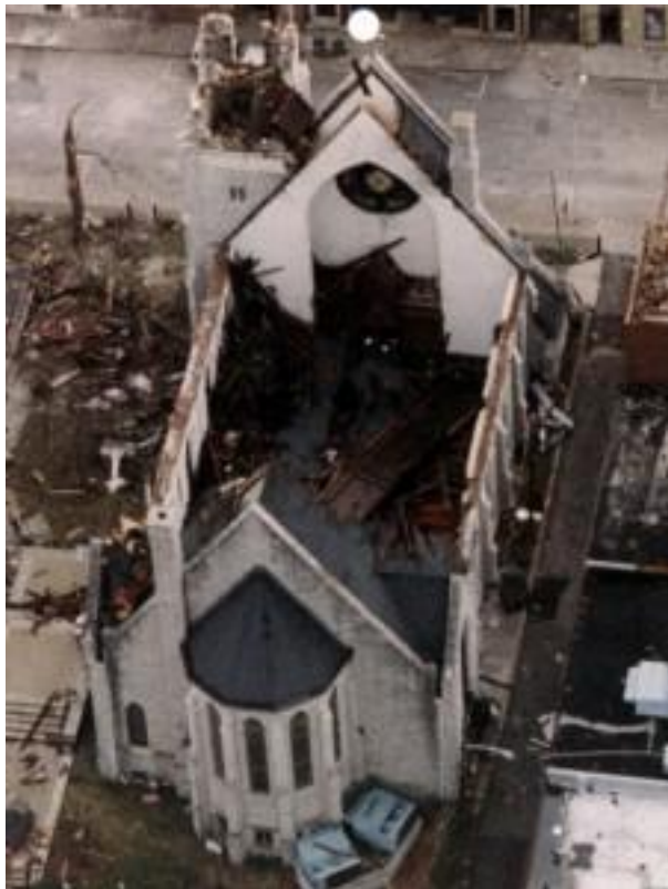
After tornado January 1999
